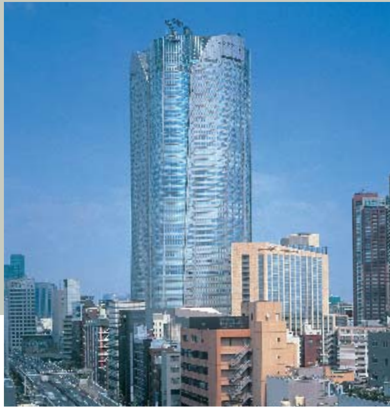
Yokohama's construction sealants were used in the 54-floor Roppongi Hills Mori Tower in Tokyo.
