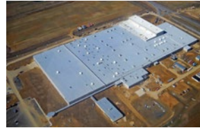
Truck and bus tire plant under construction in Mississippi
