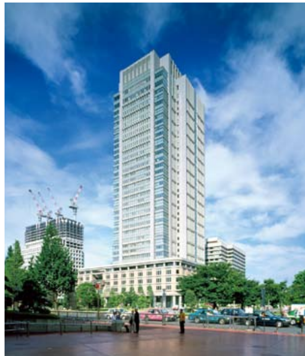
Sealants supplied by Yokohama protect the recently rebuilt Marunouchi Building, a Tokyo landmark that stands the city's flagship train station.
