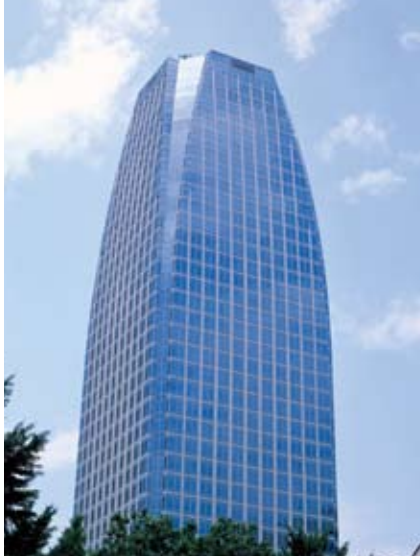
Reliable sealing. Sealant supplied by Yokohama renders service in the 42-story Mori Tower at the Atago Green Hills complex, in Tokyo. That building has captured attention for its advanced anti-seismic protection.
