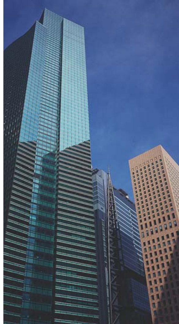
Numerous high-rise buildings at Shiodome Shiosite, a large residential and commercial urban redevelopment project in Tokyo's Minato Ward, incorporate Yokohama building sealants.
